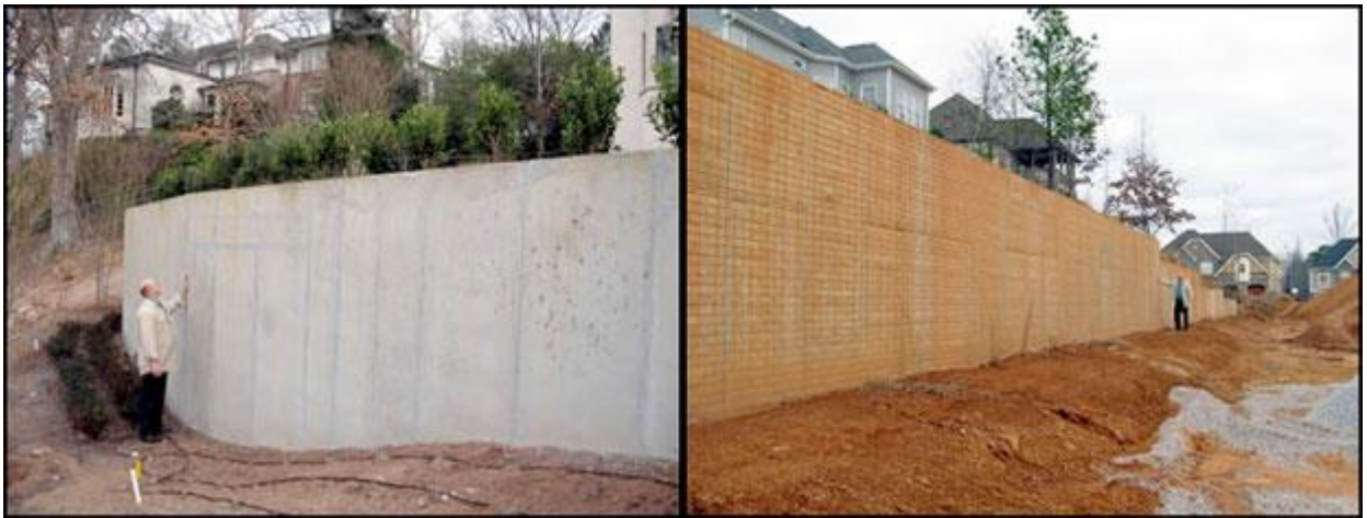
Figure 20 : Photographs of Typical Concrete Retaining Walls (Engineering Tech, 2015)
