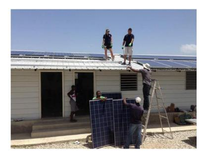
Figure 15: Typical solar panel installation on a sloped roof (Circelli, 2013)
