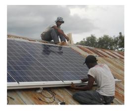
Figure 7: Solar panels being installed (Solar Electric Light Fund, 2013)
