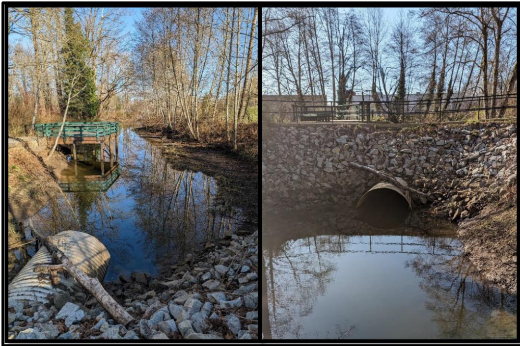
Figure 5: Simms Creek study site. One of the pool features (left), and the new “fish friendly” culvert as seen at high tide when fish can pass in between the pools and the Courtenay River (right).
