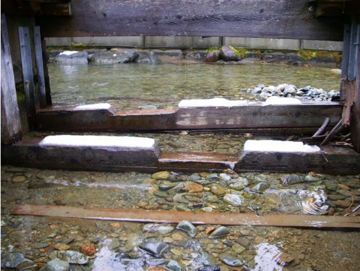
Figure 7: Sediment infilling of fish way baffles between Blackcomb Creek and Lost Lake. Photo by Jen Carter. April 6, 2005.
