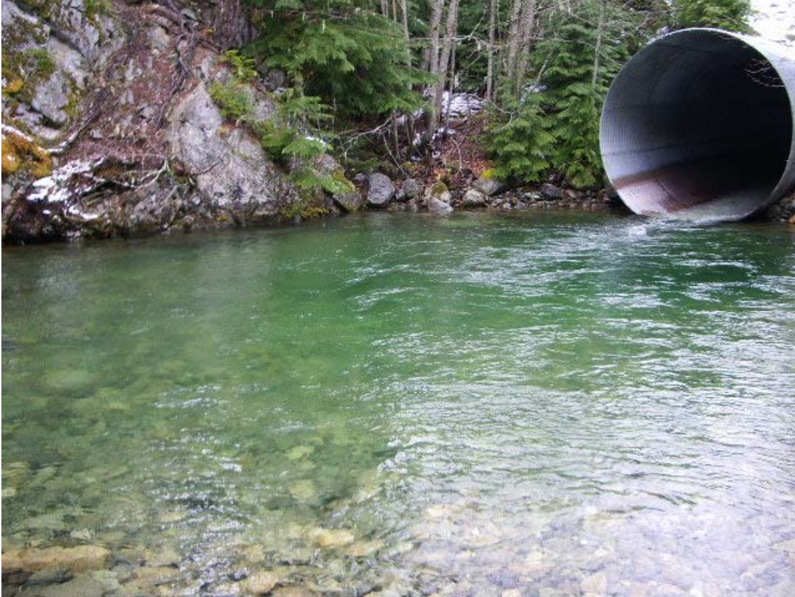
Figure 6: Twentyone Mile Creek culvert beneath Rainbow Road. Photo by Zac Semeniuk. April 8, 2004.
