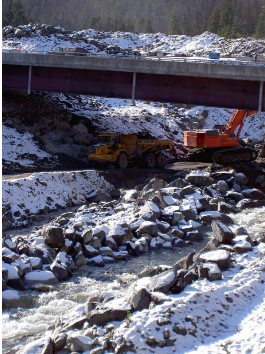
Figure 10: Construction occurring within the Rutherford Creek channel. Photo by Zac Semeniuk. November 3, 2004.
