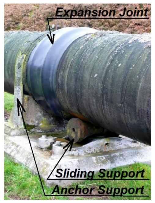
**Problem 4:** An 8" Schedule 40 straight length of steam pipe is fitted between two fixed anchor supports with no allowance for expansion. If the compressive stress in the pipe must be limited to 50.7 ksi when in operation at 430°F, determine the initial tensile stress that must be applied during installation at 60°F. What equivalent tensile force is required by this cold-springing installation?
