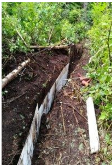
Figure 15 Photo of groundwater dam construction at the northeast corner of Camosun Bog in June 2019. Shown are sheets of corrugated plastic hammered into the upper peat layer.
