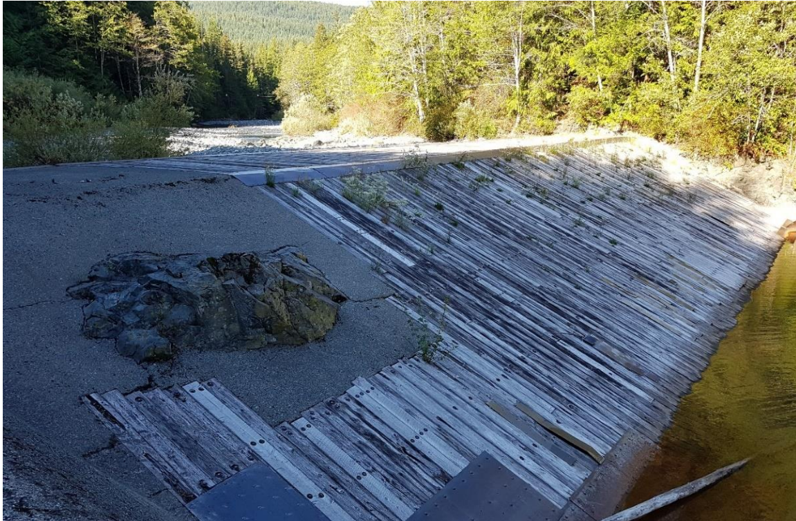
Figure 18. Photograph showing artificial elevation gradient between the upstream and downstream sections surrounding the Salmon River diversion. Upstream gravel berm is level with top of diversion. Photo taken by S. Byrne August 29, 2017.
