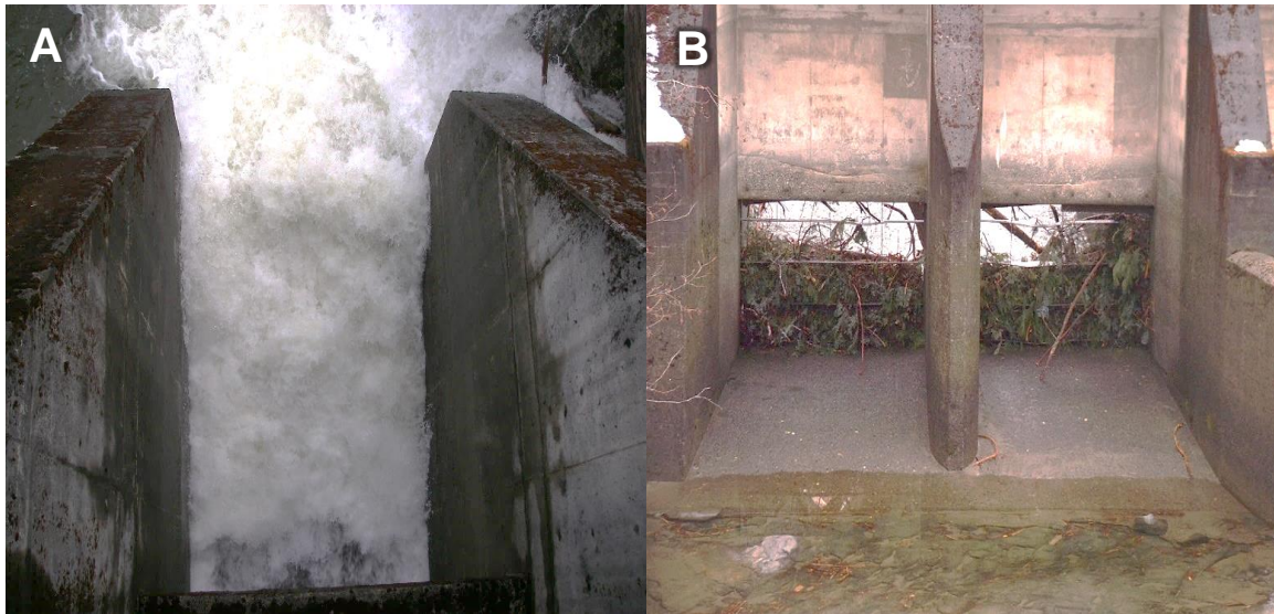
Figure 19. Photo representations of fish passage conditions for salmonids. A) The Salmon River diversion undersluice gate during diversion operation. B) Small wood debris building up within canal inhibiting salmonid migration. Photos taken by BCCF on April 6, 2006.
