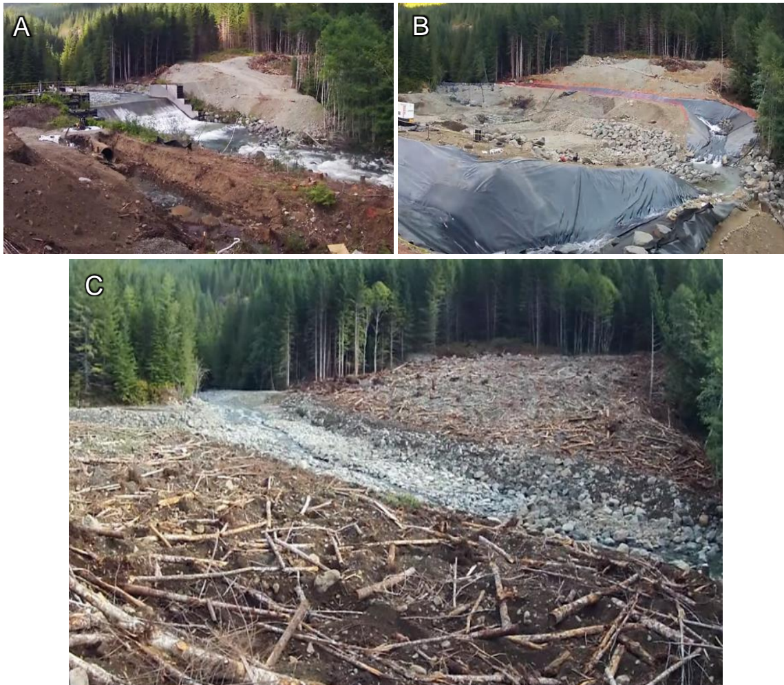
Figure 20. Progression of restoration efforts on BC Hydro's Heber River diversion 2012. Restoration involved dam and penstock removal, channel reconstruction, and riparian treatment (BC Hydro 2012).
