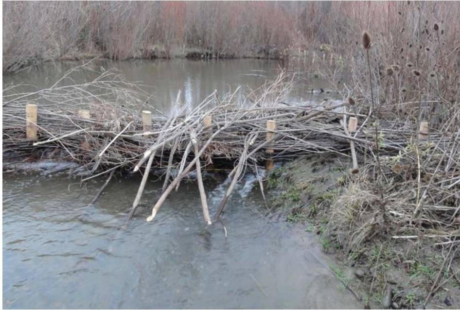
Figure 4-3: Natural flow control structure made to mimic the functions of a beaver dam (Pollock et al., 2012)
