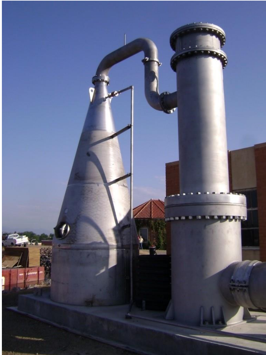
Figure 17. Example of a Speece Cone built for Marston Reservoir, Denver, Colorado. Image from Dominik (2017)
