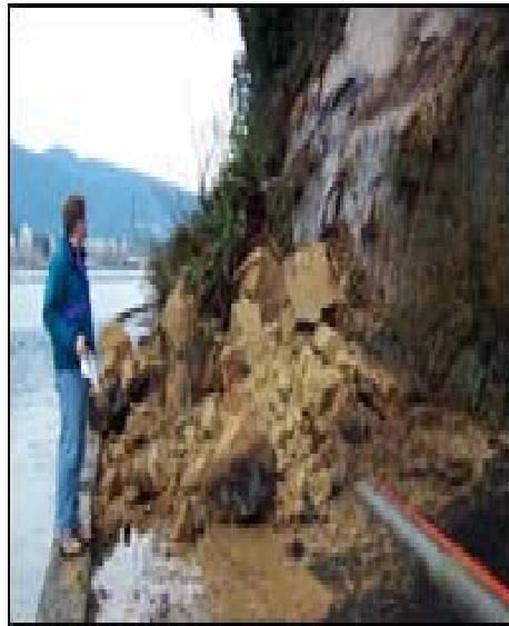
Figure 10. Mudslides due to heavy precipitation on the west side of the Stanley Park seawall. (source: Vancouver Parks Board of Recreation, 2004).
