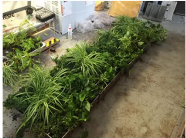
Figure 15: Living walls were first planted and placed on a horizontal surface (Daneshpanah, 2019).
