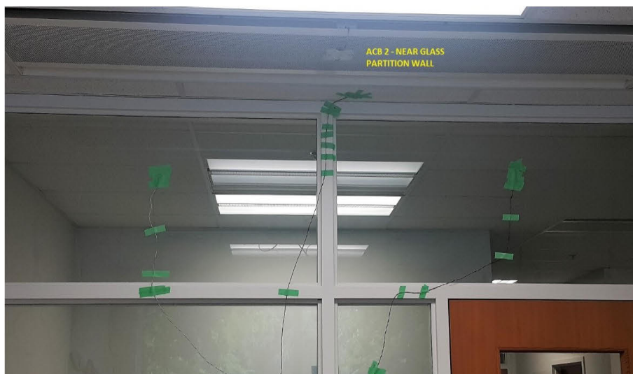
Figure 7.8 – Active Chilled Beam 2 (ACB 2) Installed near the Glass Partition in the Ceiling
