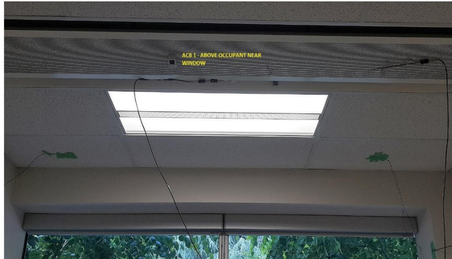
Figure 7.9 – Active Chilled Beam 1 (ACB 1) Installed near Window in the Ceiling
