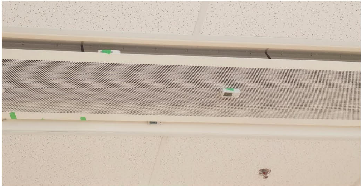
Figure 7.21 – Placement of HOBO for Discharge and Induced Air Temperature Measurement
