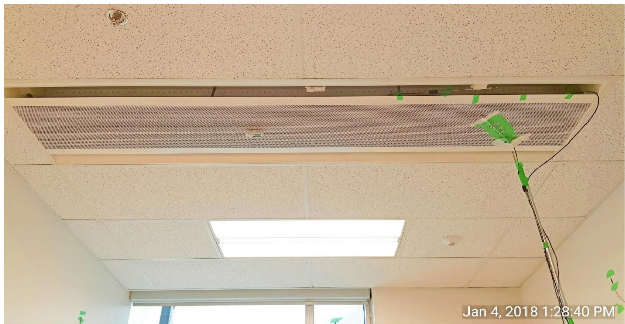
Figure 7.4 – Active Chilled Beam installed in the Ceiling
