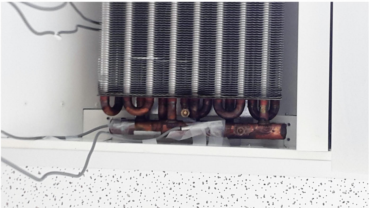
Figure 7.30 - Supply and Return Water Temperature Measurement
