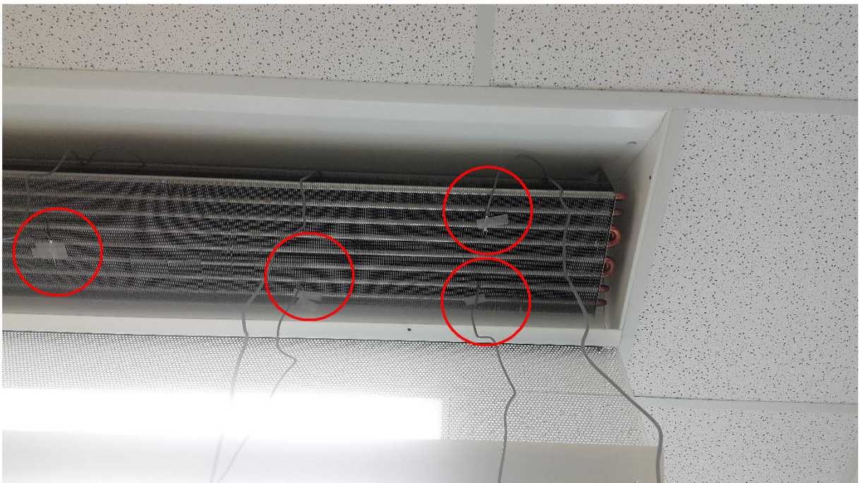
Figure 7.32 – Placement of External Temperature Sensor at Coil Surface
