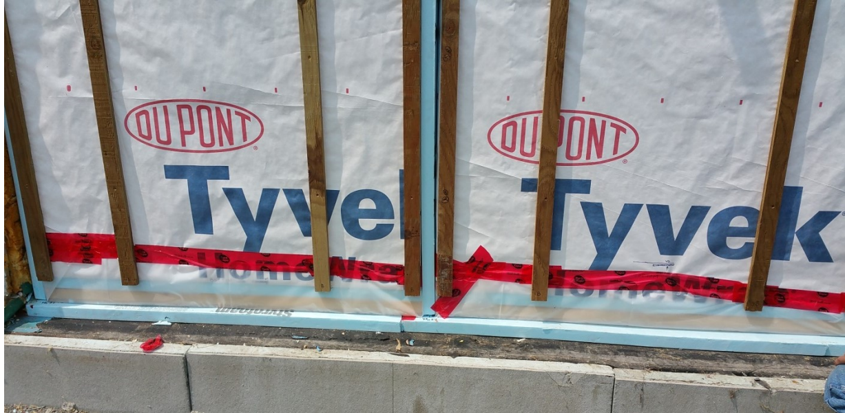
Figure 56- Walls Installed with 2" XPS Insulation between Panels
