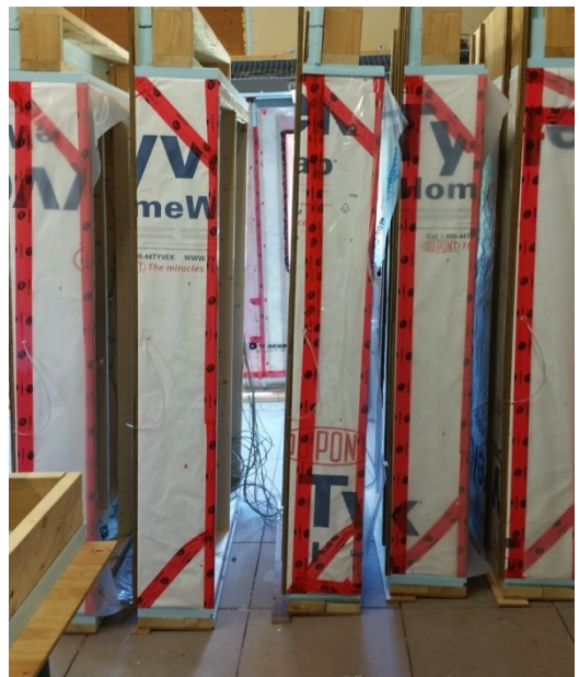
Figure 51- Wall Panels Ready for Installation
