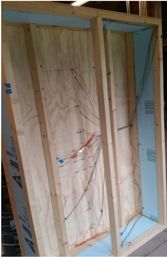
Figure 49- Walls ready for WRB and Polyethylene
