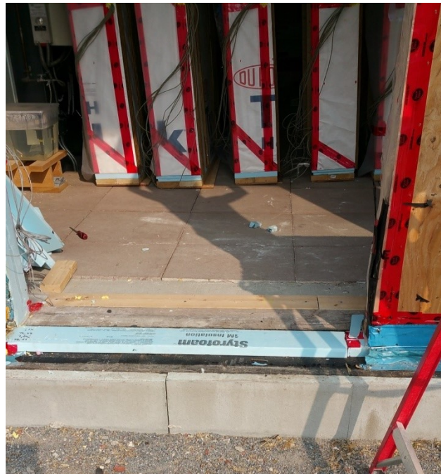
Figure 52- XPS Thermal Insulation on the bottom of walls
