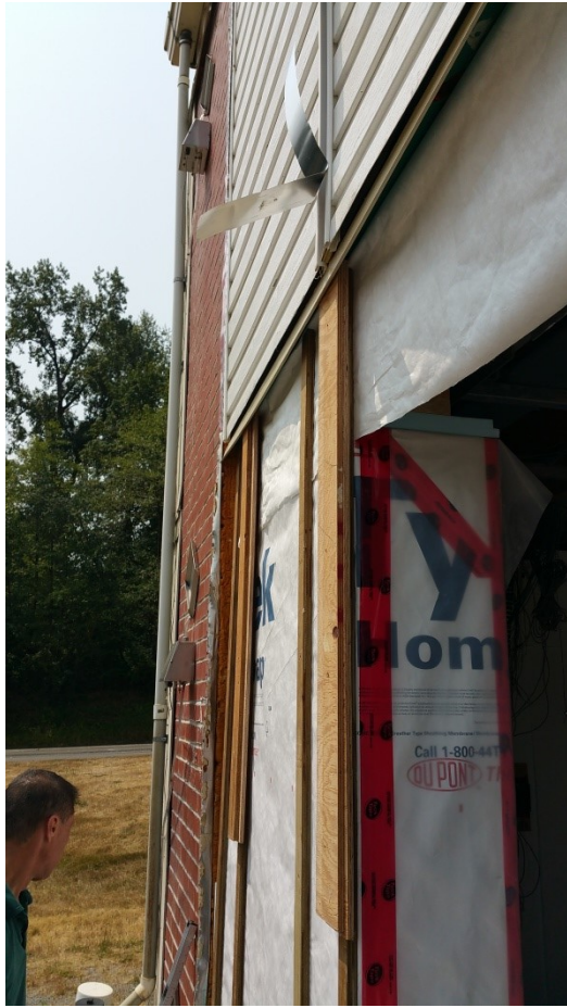
Figure 55- Flashing and Waiting WRB Overlap for Water Shedding of Siding
