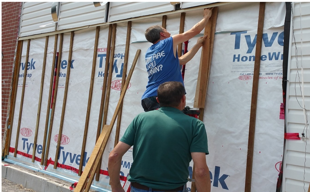
Figure 57- Attaching Wood Strapping
