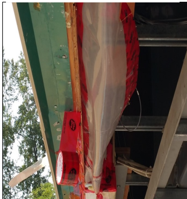
Figure 53- Maintaining Air-Tightness Continuity for Building Envelope and Wall Panels
