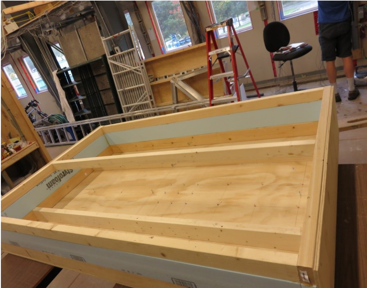
Figure 45- Wood Frame Wall Construction
