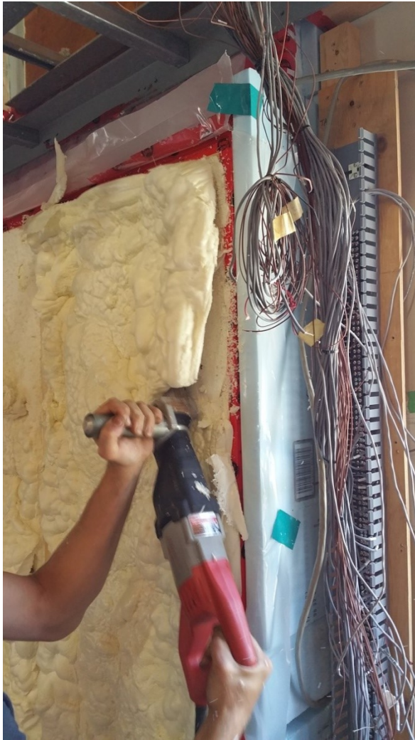
Figure 62- Sprayfoam Trimming
