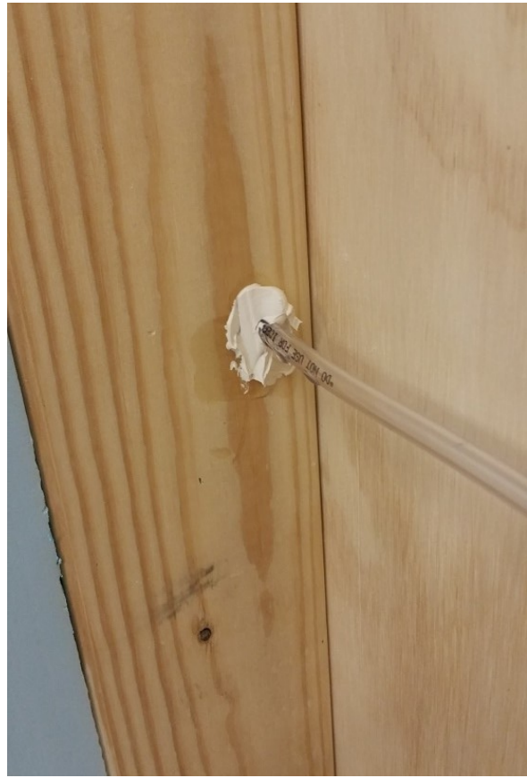
Figure 50- Water Tube through Exterior Stud
