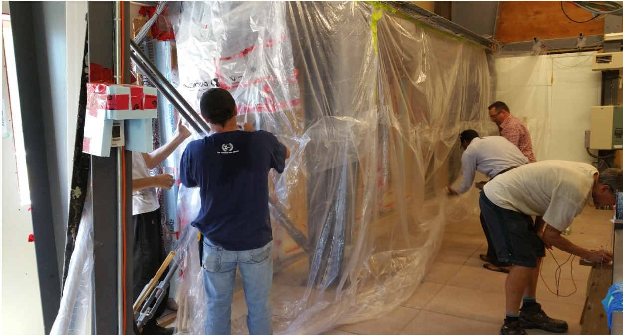
Figure 59- Application of Wet Cellulose in Isolated Chamber
