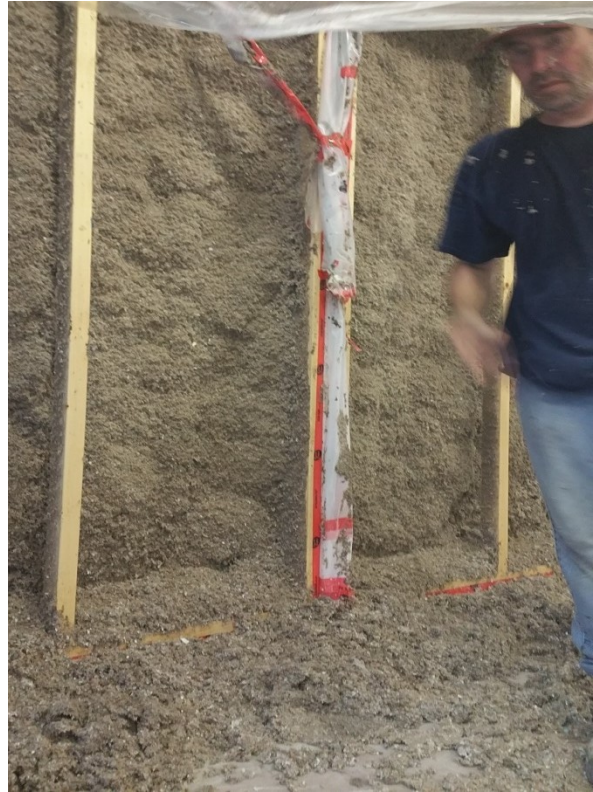
Figure 58- Wet Cellulose Application Process- First Layer
