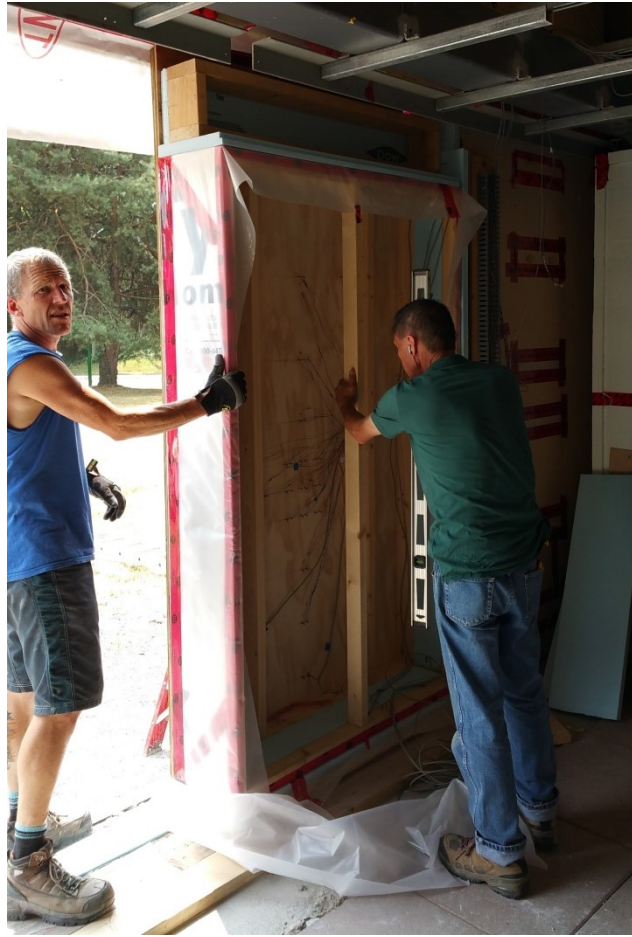
Figure 54- Walls Erecting in Building Enclosure
