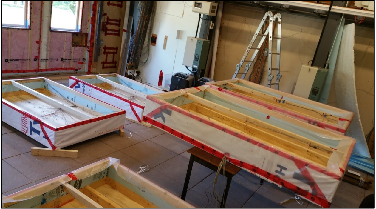
Figure 33- Wall Panels- Encased in Vapour, Air and thermal barrier in the perimeter (photo by author)
