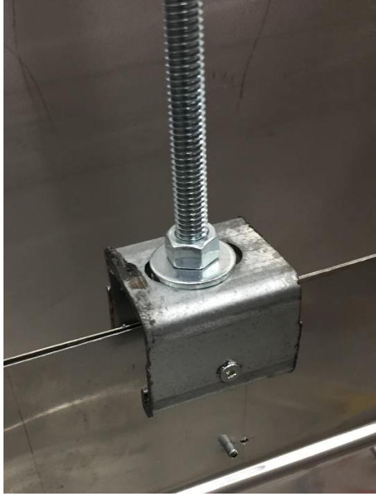
Figure 4.22 - Plate Support Connection
