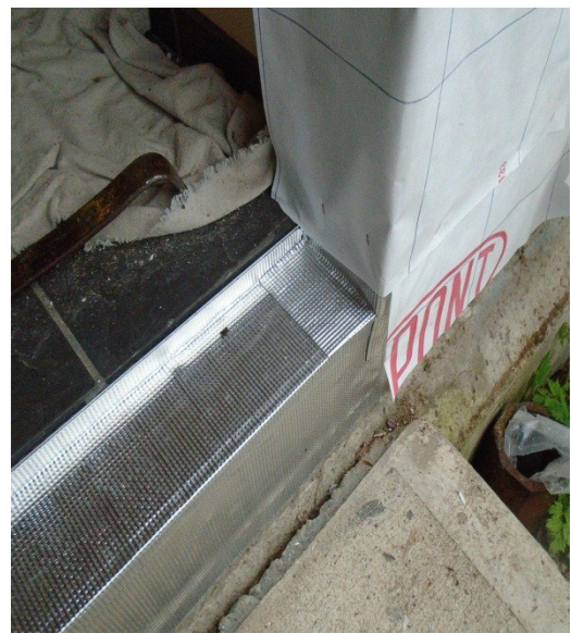
Waterproofing at the Sill
