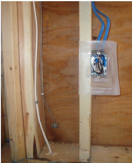
Figure 36: Moisture content sensor below bathroom window near electrical outlet
