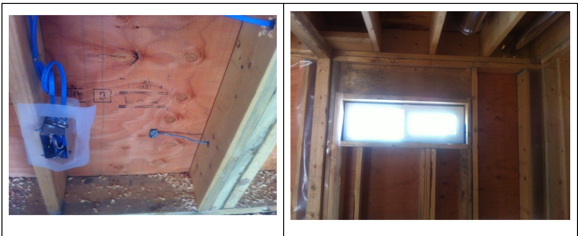
Figure 18: Polypan at electrical outlet and poly pre-stripping at the wall.
