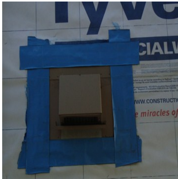
Waterproofing detail around a vent
