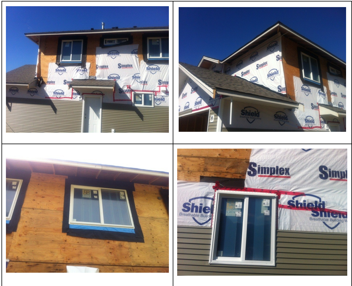
Figure 14 Exterior walls with sheathing membrane and vinyl cladding
