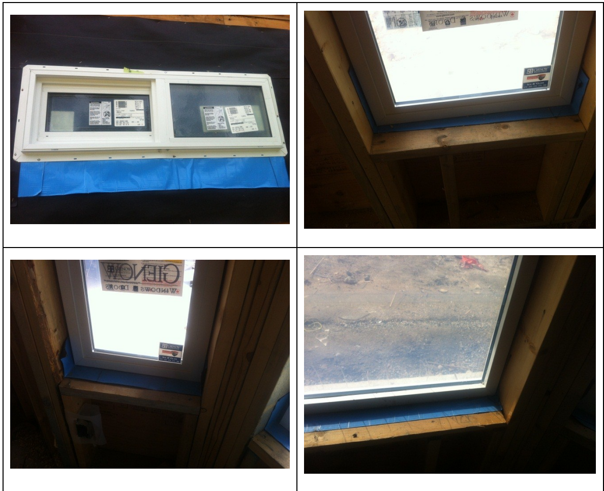
Figure 19: Installation of SAM at window sills.
