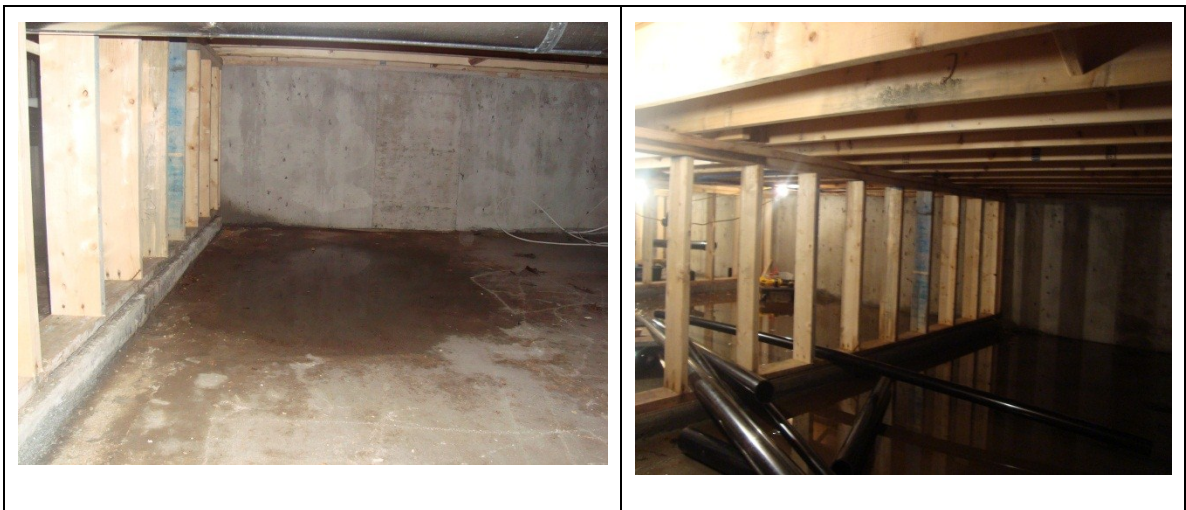
Figure 22: Construction moisture on crawlspace floors
