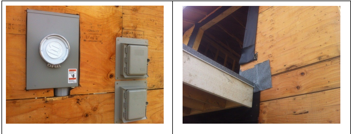
Figure 16: Photo1 shows the meters are neither pre-stripped with membrane nor waterproofed Photo 2 presents the balcony saddle detail
