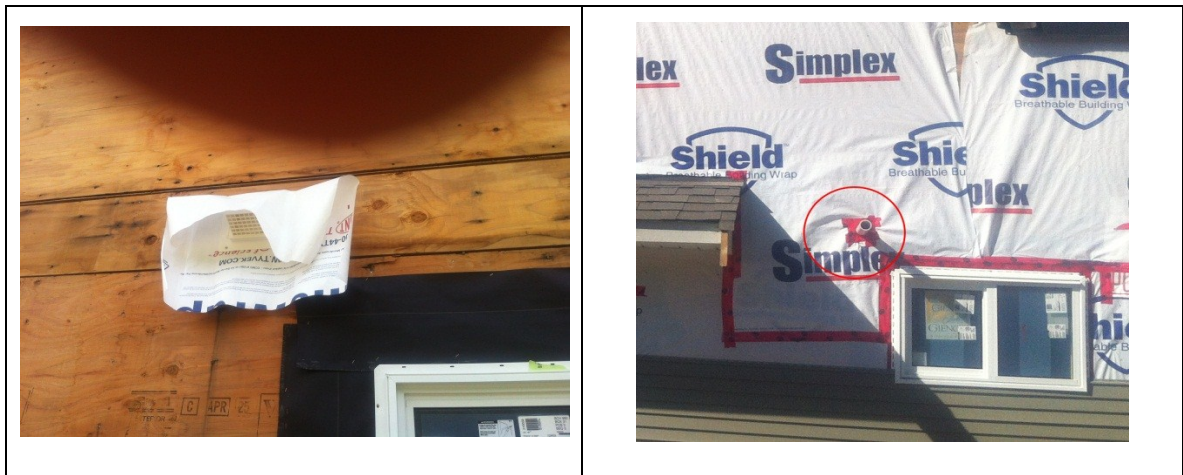
Figure 15- Photo 1 shows the exhaust penetration pre-stripped with sheathing membrane Photo 2 shows the pipe penetration stripped and sealed with red tape only
