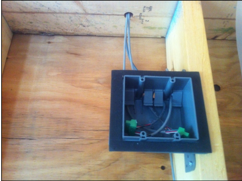
Data Acquisition Unit Box (Sensors are terminated in the box for connections to Data Acquisition Unit)
