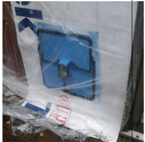
Detail around an electrical outlet
