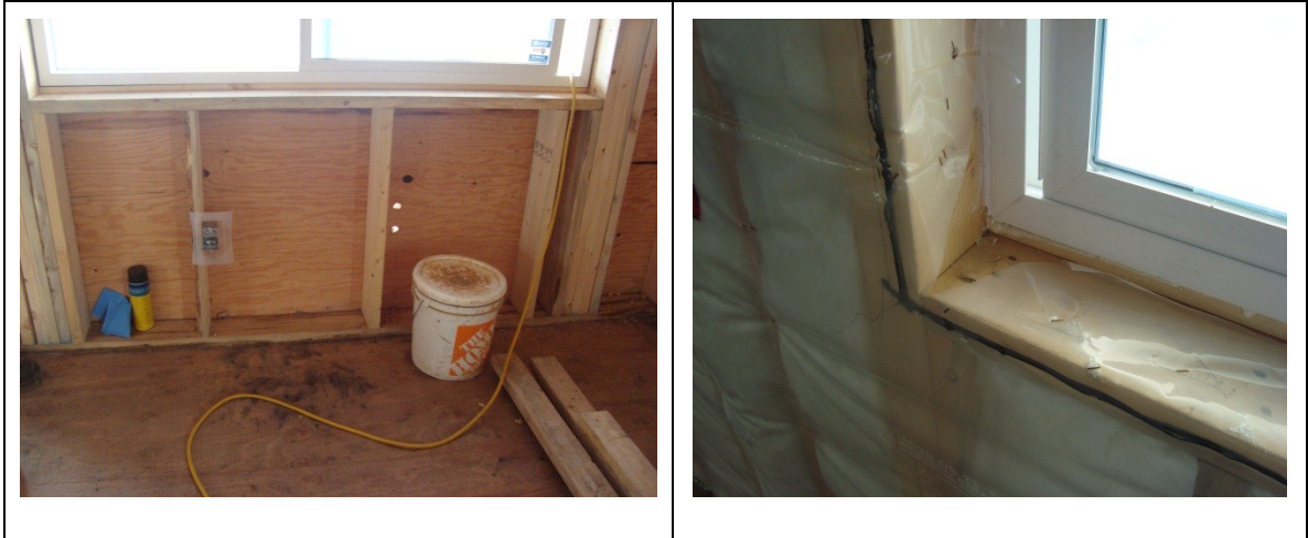
Figure 20: Window sill detail deficiency as there is no weatherproofing (SAM) installed at the sill on three windows
