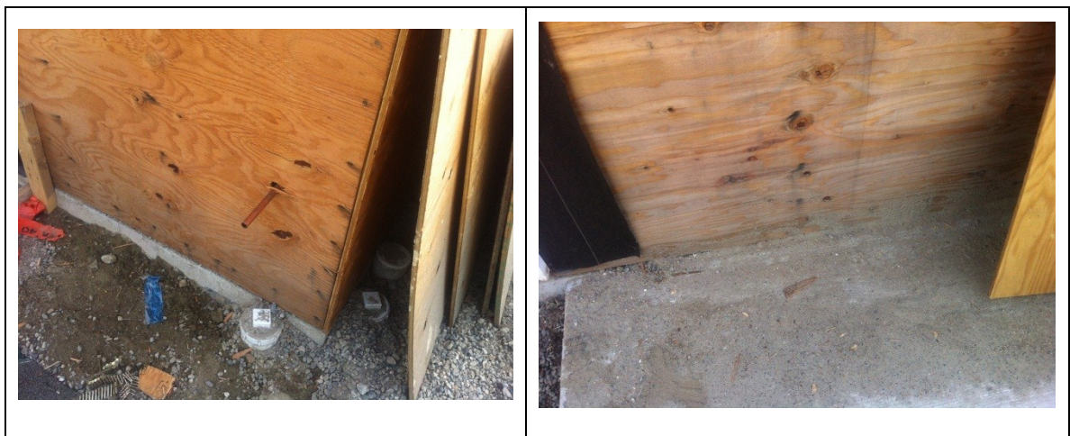
Figure 17: Capillary break missing at the concrete to wood transition
