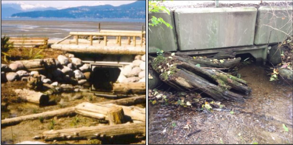
**Figure 18:** The lower reaches of Spanish Bank Creek have been filled with sediment. Installed in 2000, the concrete box culvert pictured above is 6 m long, 1.2 m tall, and 1.8 m wide (left; Hollick-Kenyon, 2002). After 16 years only a fraction of the culvert is passable due to build-up of sediments (right; Reynolds, 2016).
