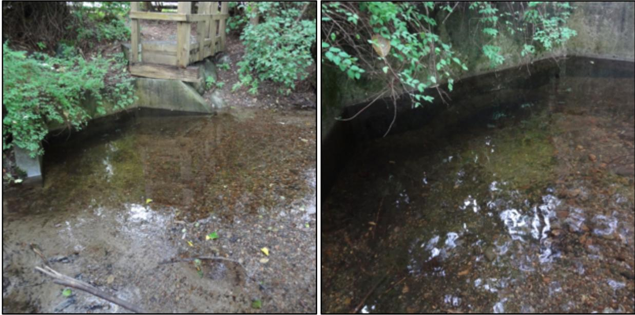
**Figure 19:** A pre-cast concrete headwall was installed at Spanish Bank Creek. The pre-cast concrete headwall is located at the north end of the wood stave culvert that spans under NW Marine Drive (left). Accretion of sediment has filled in the lower reaches of Spanish Bank Creek, thereby impeding flow through the wood stave culvert (right; Reynolds, 2016).
