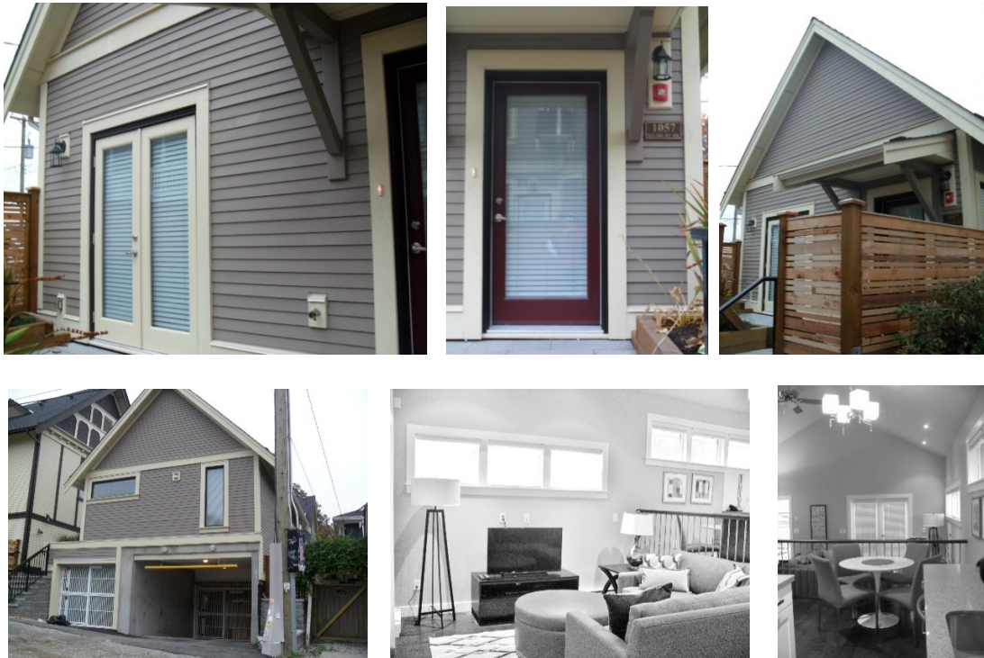
Figure 22: Aerial Google Earth image of LWH C location (first image on previous page), Test Facade C at south (second image on previous page and three on top of this page), lane side view (above left) and associated indoor space (two above right).
