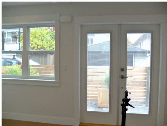
Figure 107: Very high fenestration/facade ratio on the lane side with high noise level
