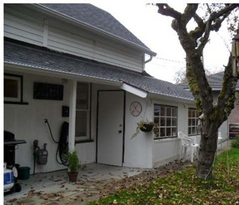
Figure 23: Aerial Google Earth image of LWH D location (first image on previous page), Test Facade D on north (second image on previous page), outdoor views (above right and above) and associated indoor space (above left).
