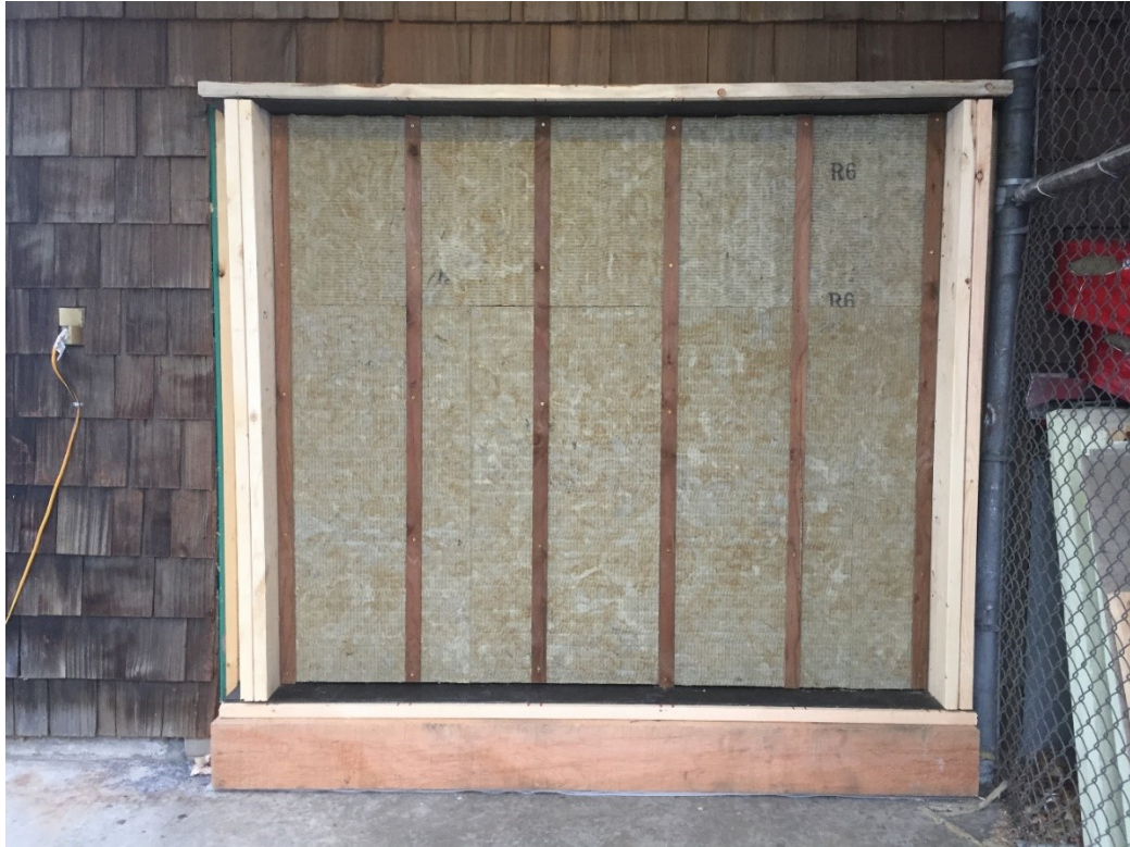
Figure D.10. Wood strapping and mineral wool exterior insulation.
