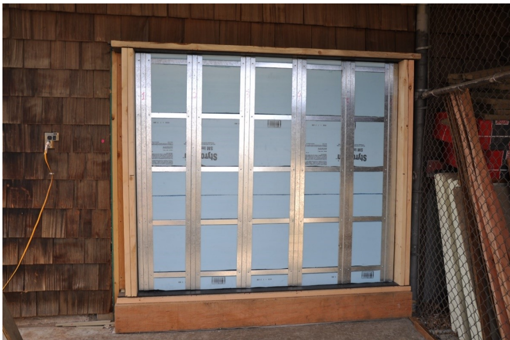
Figure D.8. Horizontal Z-girt and XPS exterior insulation.
