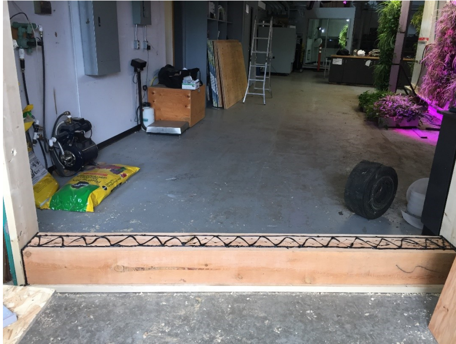
Figure E.17. Acoustic sealant applied over the 8" x 8" wood.
