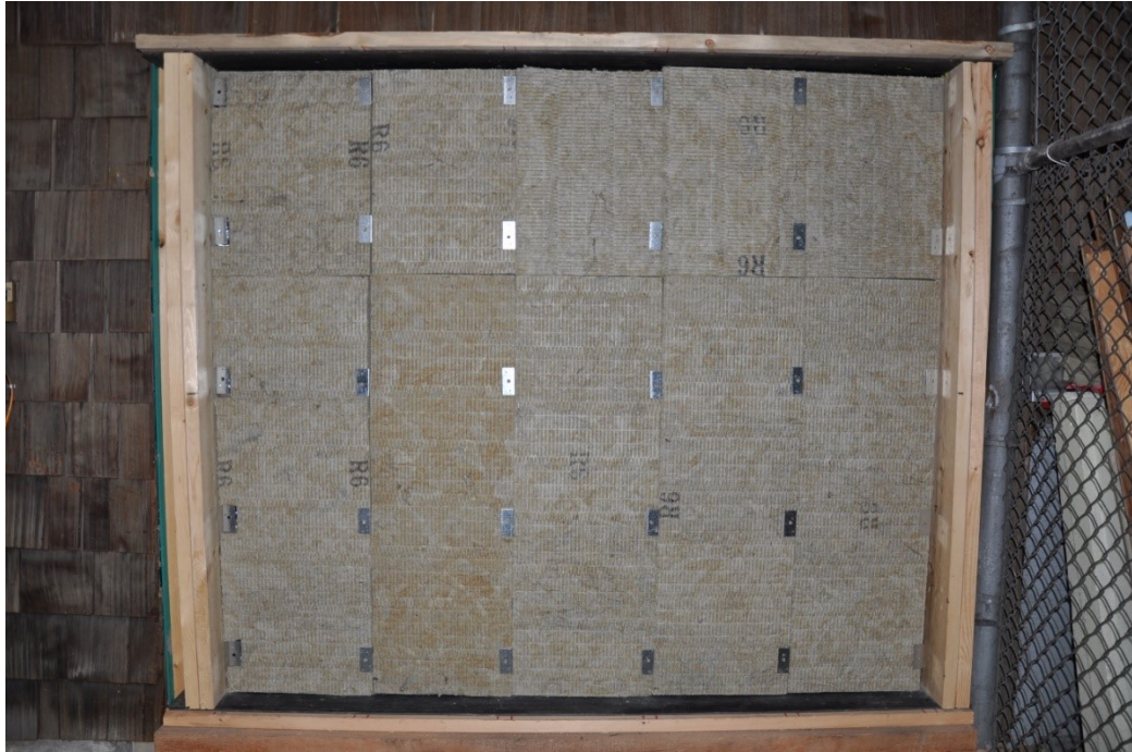
Figure D.2. Metal clips and mineral wool exterior insulation.
