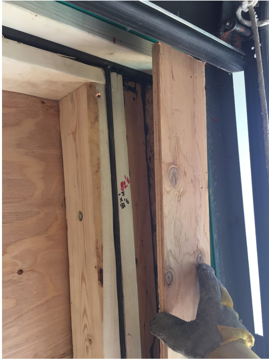
Figure E.24. Piece of wood board covering the wood filling laterally.
