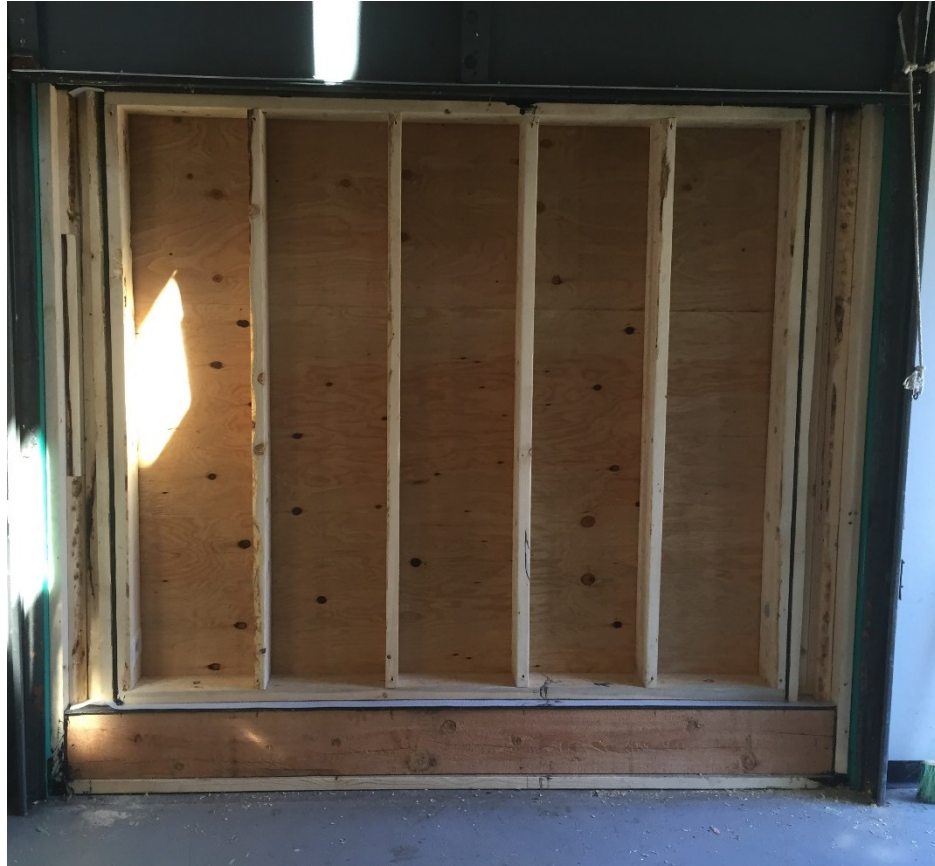
Figure E.25. Plywood sheathing over wood studs.
