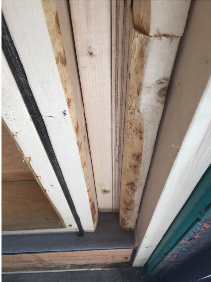
Figure E.23. Gap between the lateral wood stud and sub-frame filled with wood.
