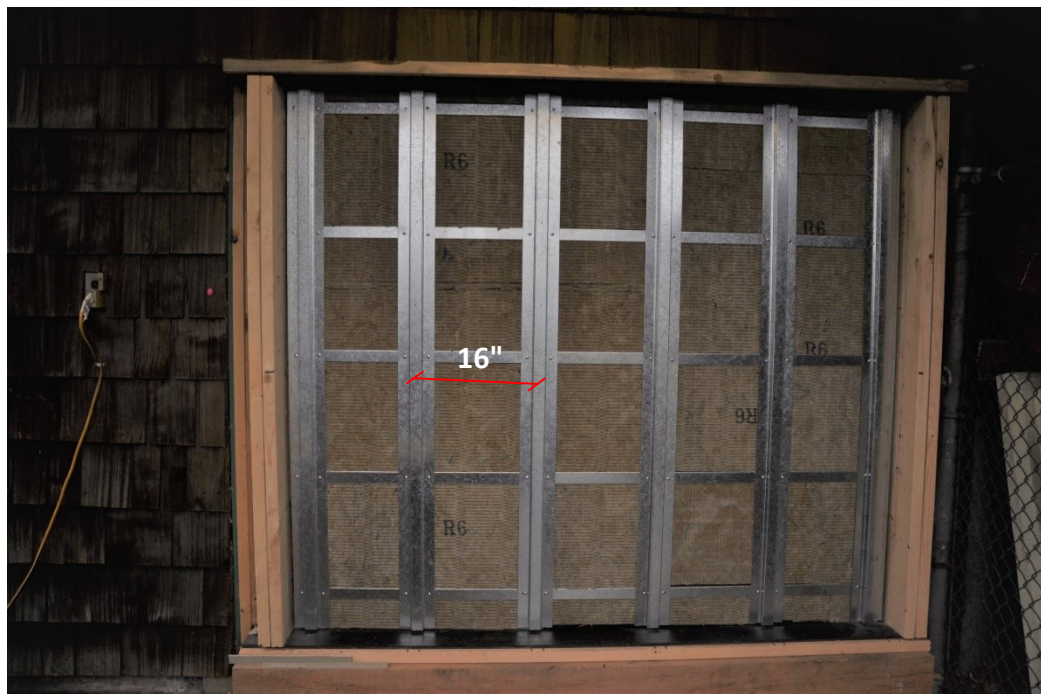
Figure D.7. Horizontal Z-girt, mineral wool, and vertical Hat-track furring.
