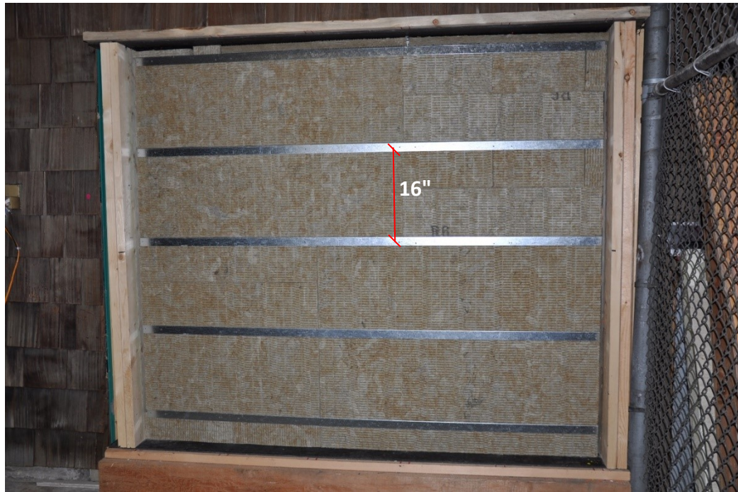
Figure D.6. Horizontal Z-girt and mineral wool exterior insulation.
