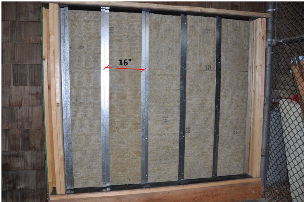
Figure D.3. Metal clips, mineral wool, and S-track steel furring.
