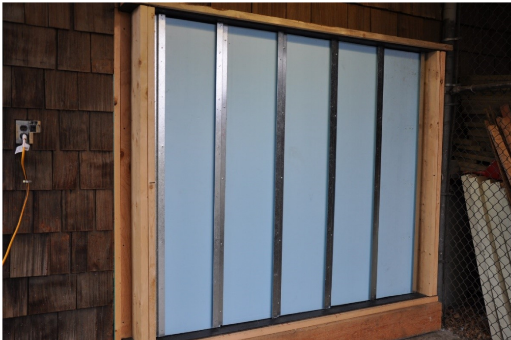
Figure D.5. Metal clips, XPS, and S-track steel furring.
