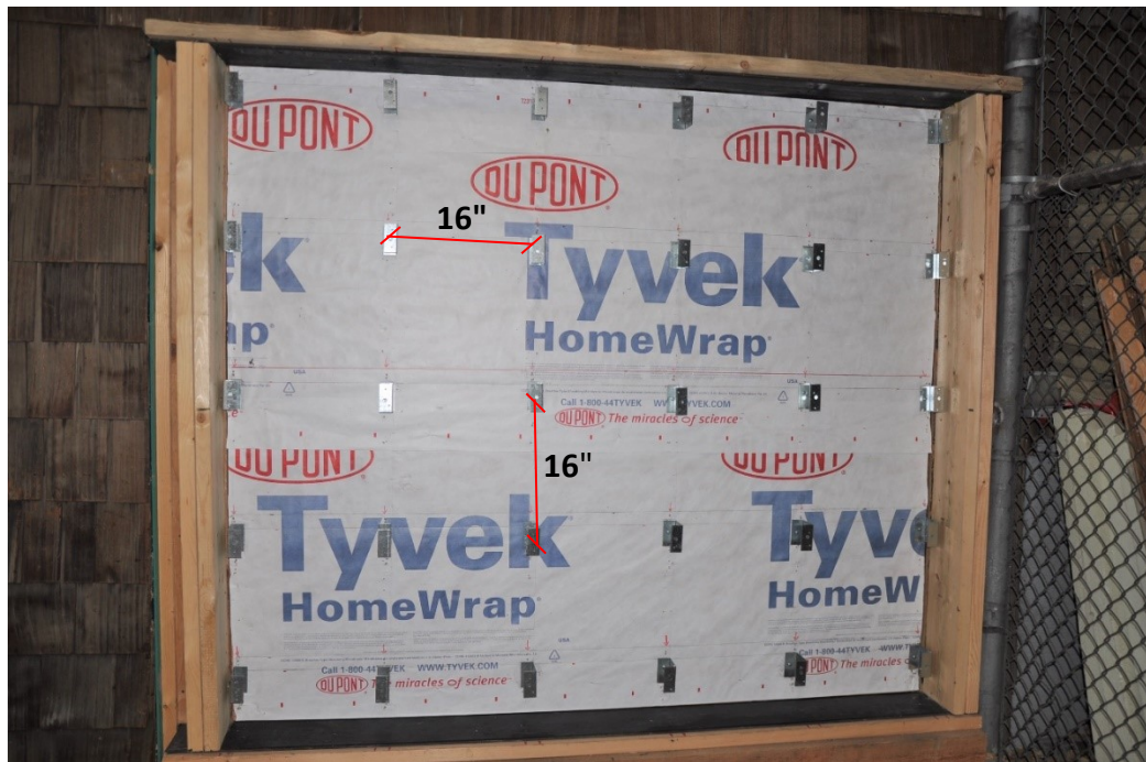
Figure D.1. Metal clips attached to the base wall without exterior insulation.
