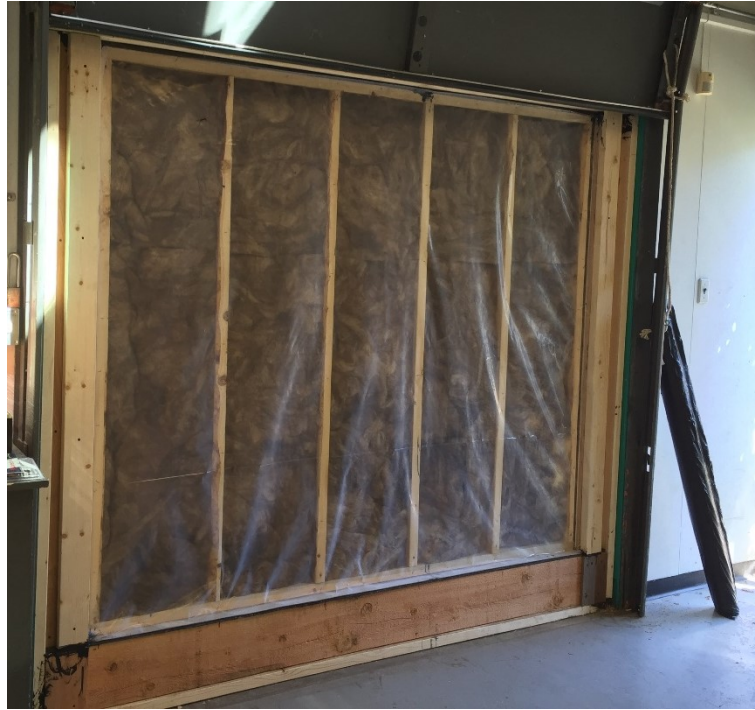
Figure E.26. Interior view of the wall with the fiberglass batts and poly membrane.
