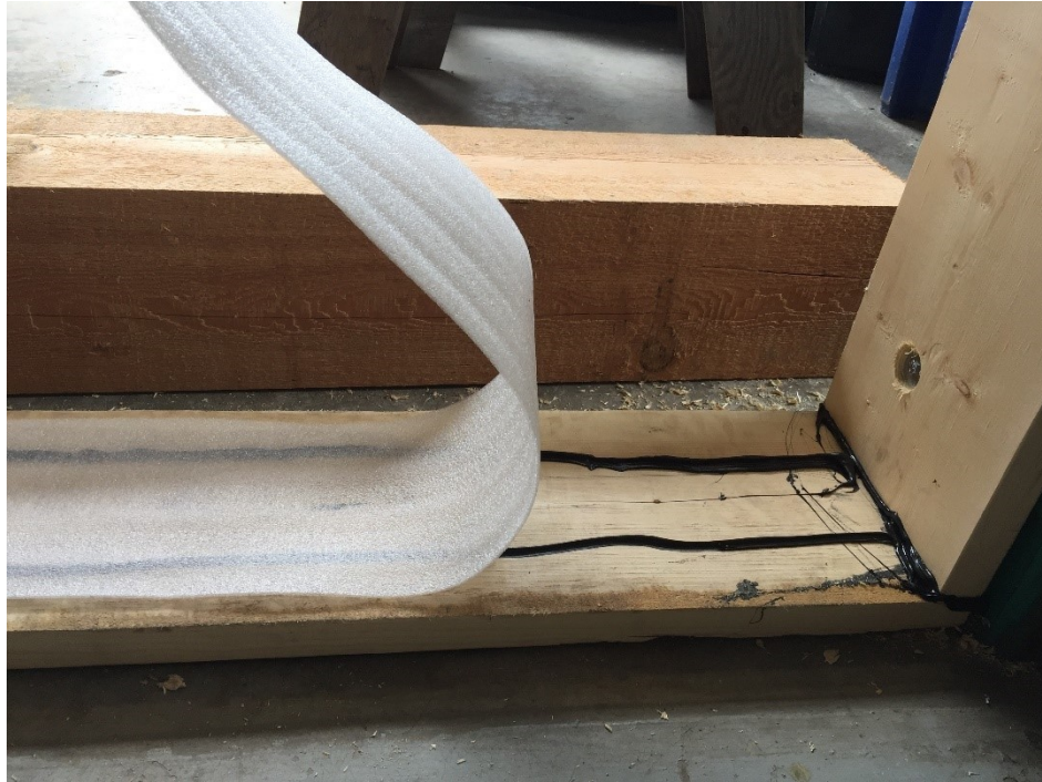
Figure E.16. Acoustic sealant and gasket over the plate.
