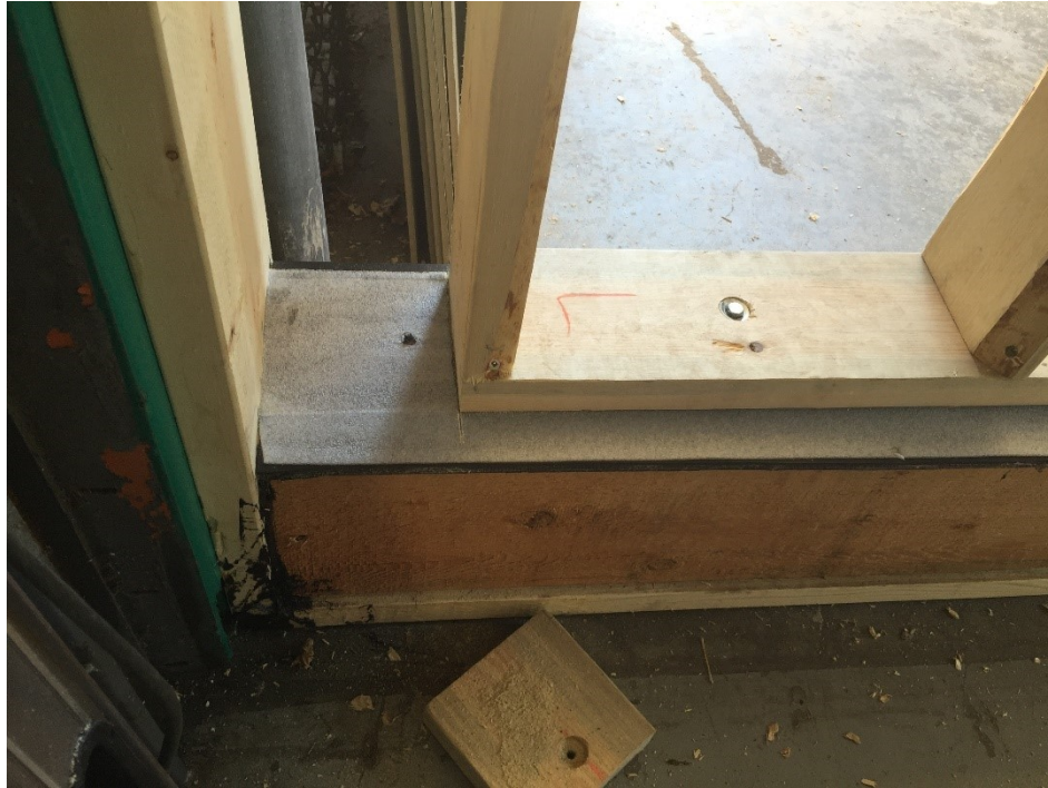
Figure E.20. Bottom plate and vertical wood studs.
