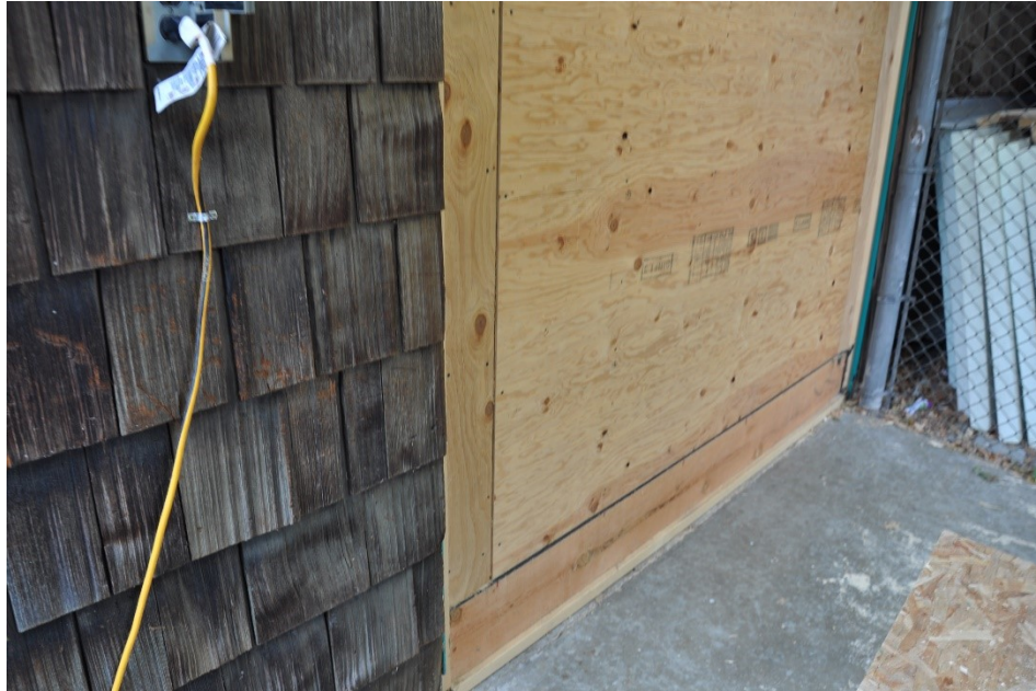
Figure E.31. Plywood sheathing flushing with the existing wall.
