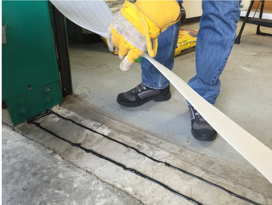
Figure E.14. Acoustic sealant and gasket application.
