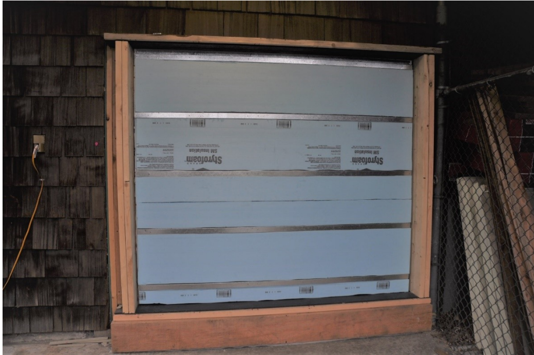
Figure D.8. Horizontal Z-girt and XPS exterior insulation.
