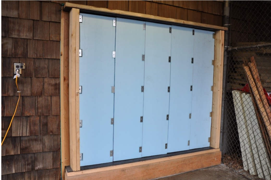
Figure D.4. Metal clips and XPS exterior insulation.
