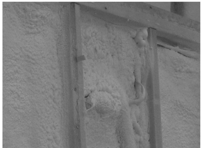
Figure 10. A photo showing the non-uniform thickness of the foam
