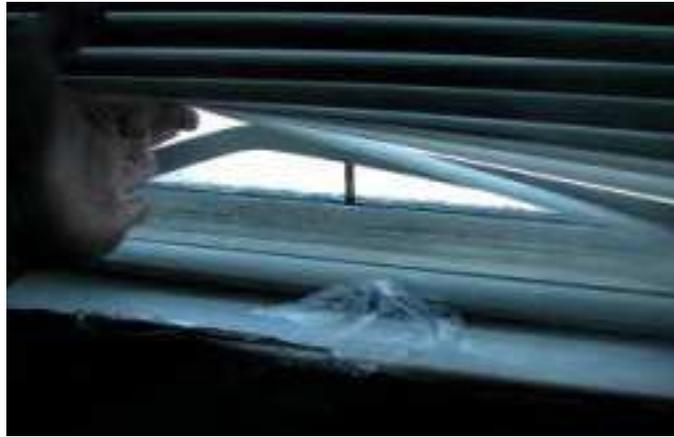
Figure 22 Excessive window condensation (Stad 2006)
