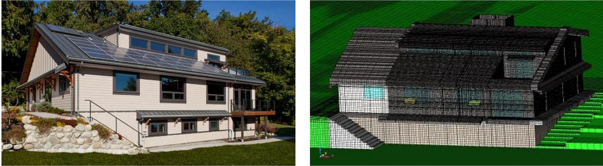
**Figure 32: Photograph of the Harmony House (left). Meshed CFD model of the Harmony House (right).**
