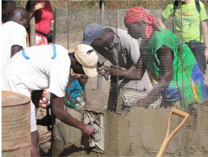
Figure 9: Community construction of a ferrocement water tank (Westra, 2010)
