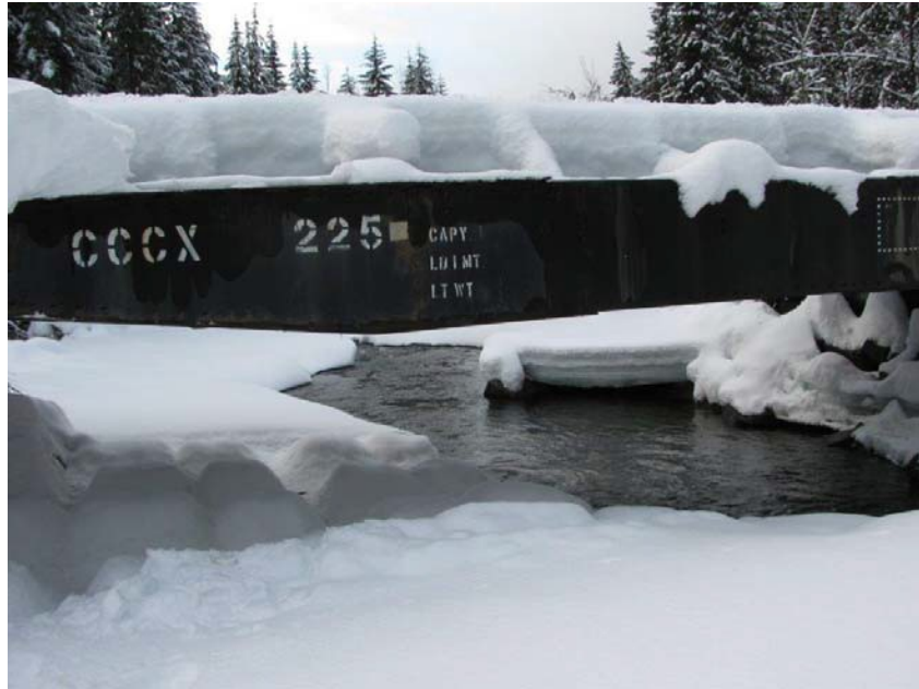
Figure 5-3. Bridge X Creek as observed from the Forestry Service Road Bridge, facing downstream.
