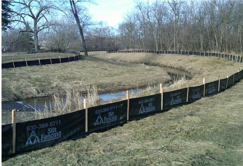
Figure 47: Typical silt fencing (Erosion and Sediment Control, 2015)
