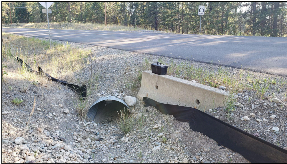
Figure 7. A traffic counter was installed on the east side of Jaffray-Baynes Lake Road beside the turtle tunnel (large culvert) from June 19 to September 5, 2023.
