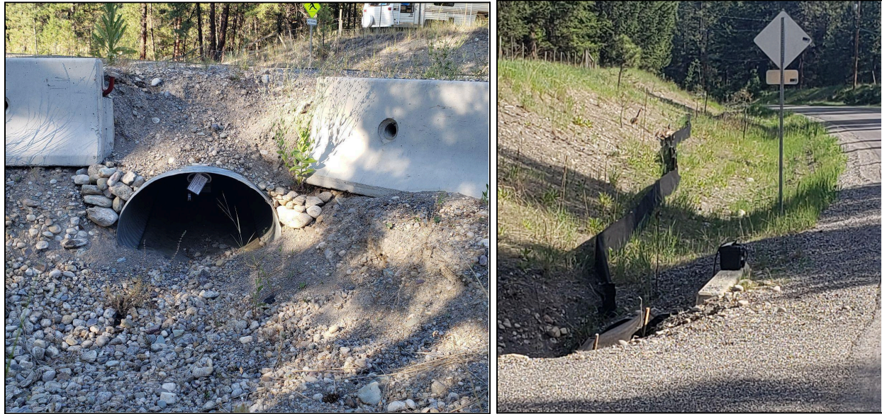
Figure 5. A culvert (turtle tunnel) and drift fencing installed at Baynes Lake, BC. Left: The Baynes Lake painted turtle tunnel installed on Jaffray-Baynes Lake Road. The white tag slightly obscured the installed wildlife camera, pointing into the tunnel. Picture was taken in 2023 facing east. Right: Drift fencing installed in 2023 along Jaffray-Baynes Lake Road to direct turtles to the turtle tunnel.
