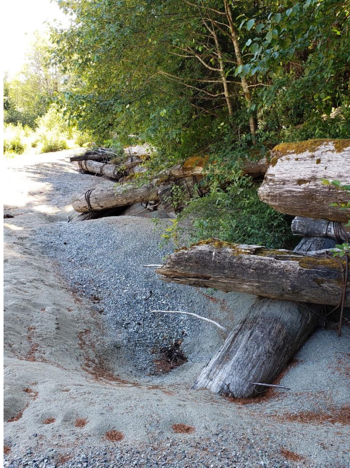
Figure 4. LWD installations along the right bank of the mainstem of Reach 1. The structures were created to armour the bank against lateral erosion and prevent side channels being engulfed by the widening mainstem. Aggradation has caused the channel to migrate away from the LWD structures, rendering them non-functional. Photograph was taken August 2 nd 2021.
