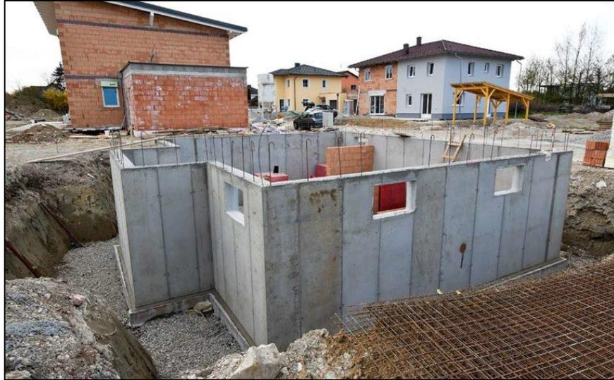
*Figure 7: Typical Basement Wall Configuration (EverDry, 2018)*
