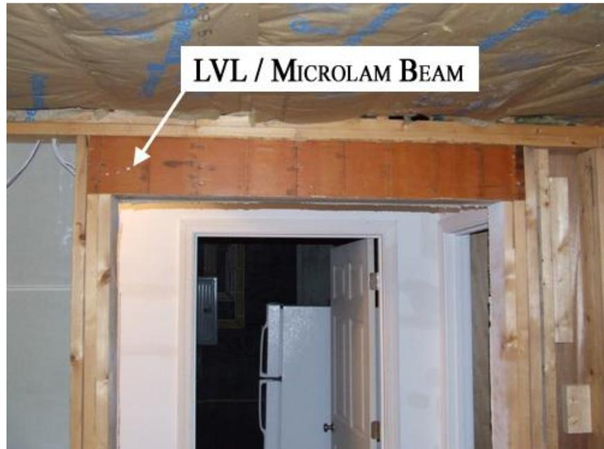
*Figure 3: Opening with a Header Beam (Fratzel, 2009)*
