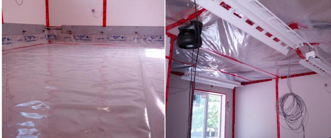
Figure 22. Concrete floor and footing (left) and gypsum board ceiling (right) were isolated from interaction with indoor air moisture by installing polyethylene sheet
