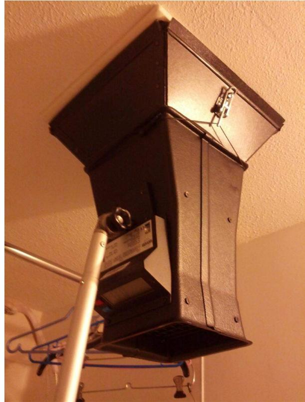
**Figure 1. Photograph of the SwemaFlow 233 unit during measurements in Suite A**
